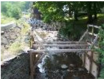
Temporary bracing holds the historic stone retaining wall.
