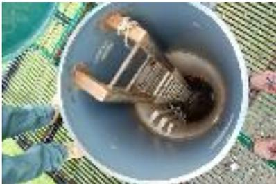
Improved manhole leads down to the lift pump.
