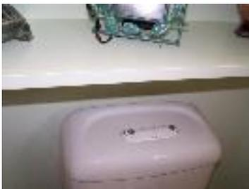
The dual flush toilet allows the user to select a 0.8 or 1.6 gallon flush.
