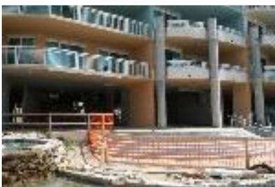
Breakaway walls on the first floor successfully blew out to save the building.
