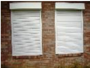
Storm shutters protected the Center from wind and debris.
