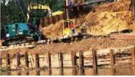
Cloverport slope stabilization.
