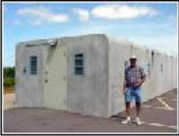
Shelters protect park residents during high-wind events
